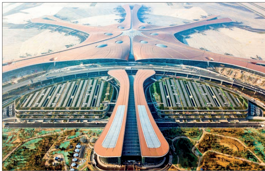
The terminal building of the Beijing Daxing International Airport in Beijing, capital of China. PHOTO: CAI YANG/XINHUA/FILE
