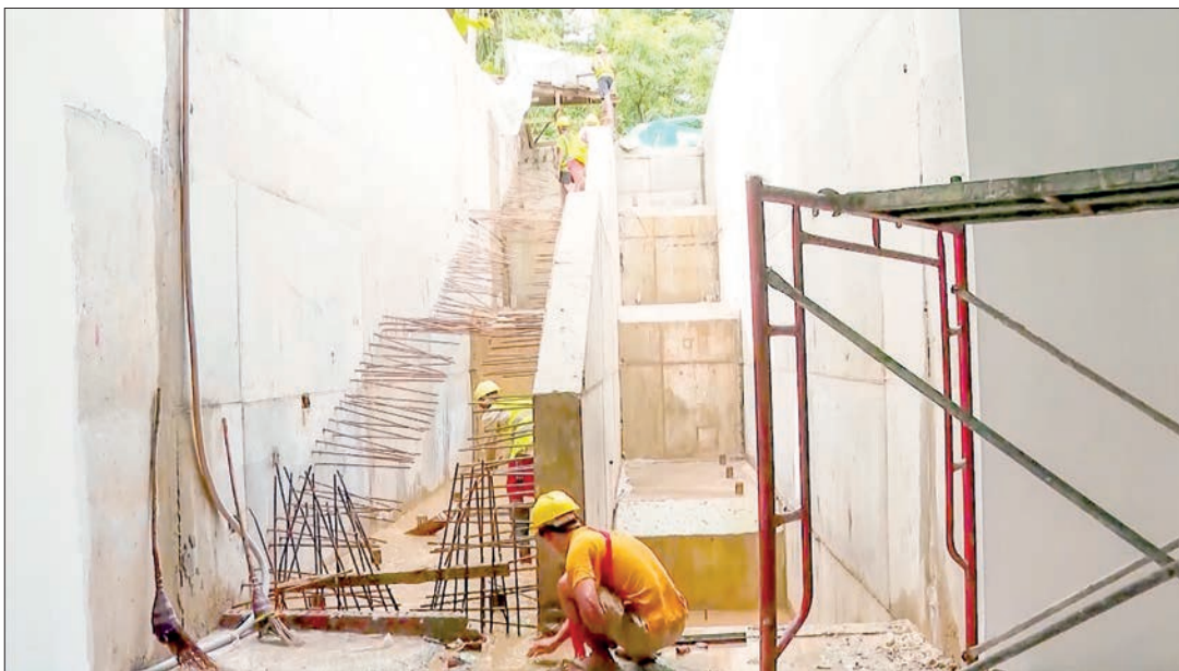
This picture captures the construction site of the underpass.
