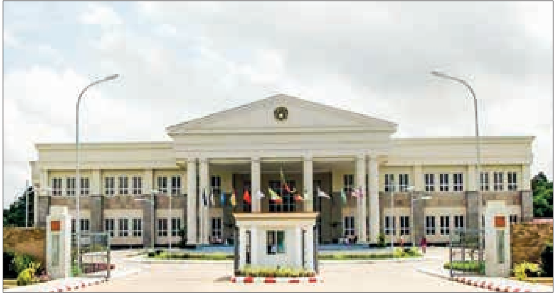
This photo shows the facade of the Myanmar Economic Bank (MEB) in Nay Pyi Taw.
