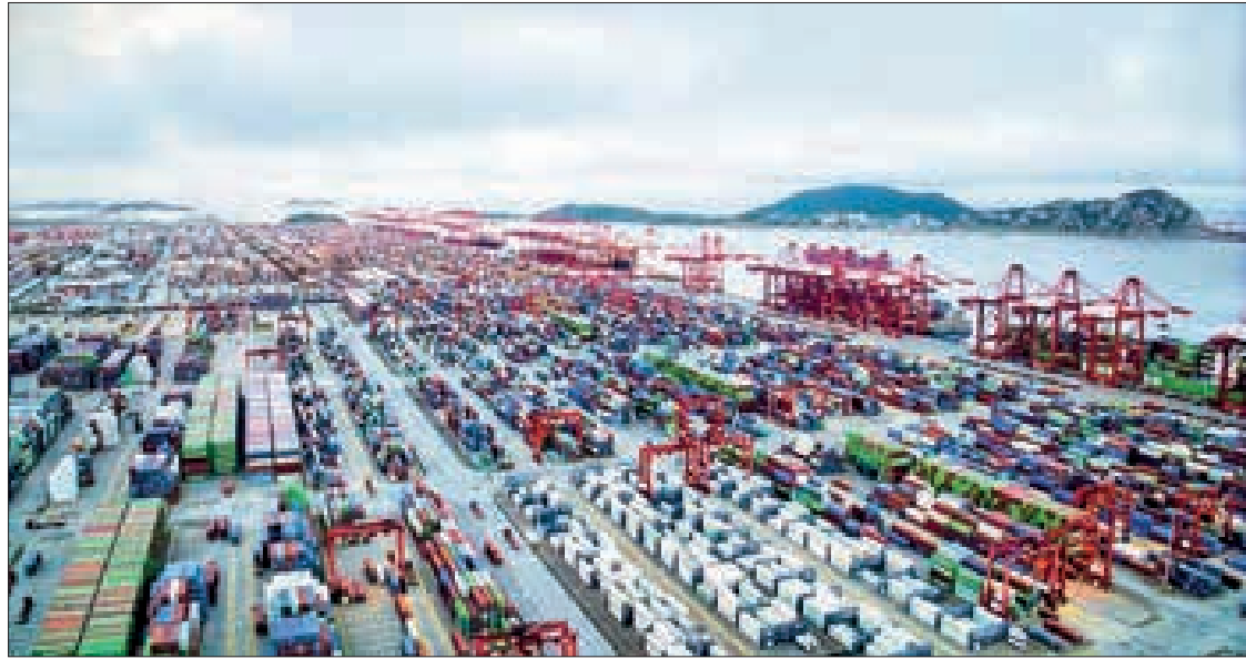
This photo taken on 17 September 2023 shows a view of the automated container terminal of Shanghai Yangshan Deep Water Port in east China's Shanghai. PHOTO: WANG YIMING/XINHUA
