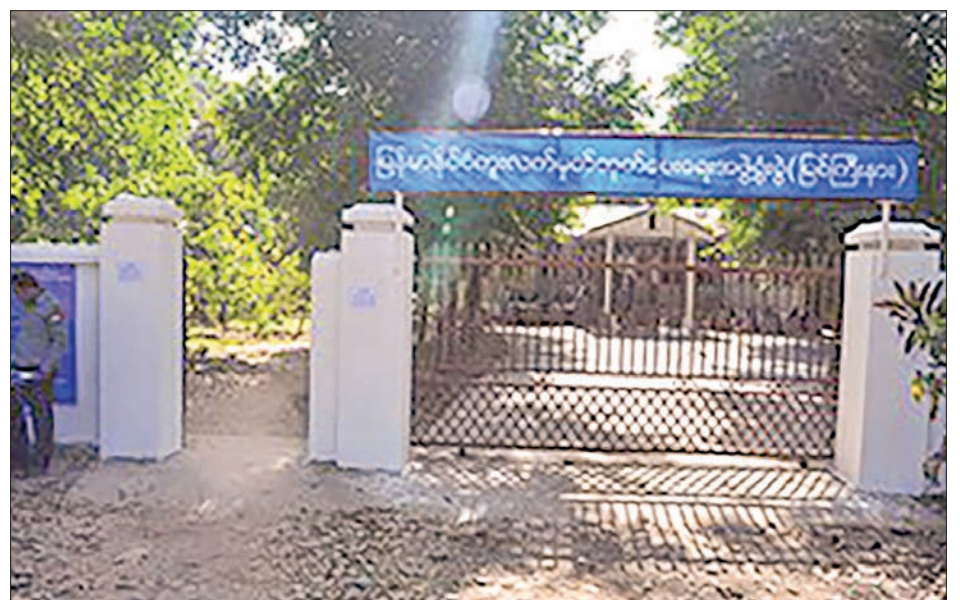
The facade of the Myanmar Passport Office (Myitkyina).
