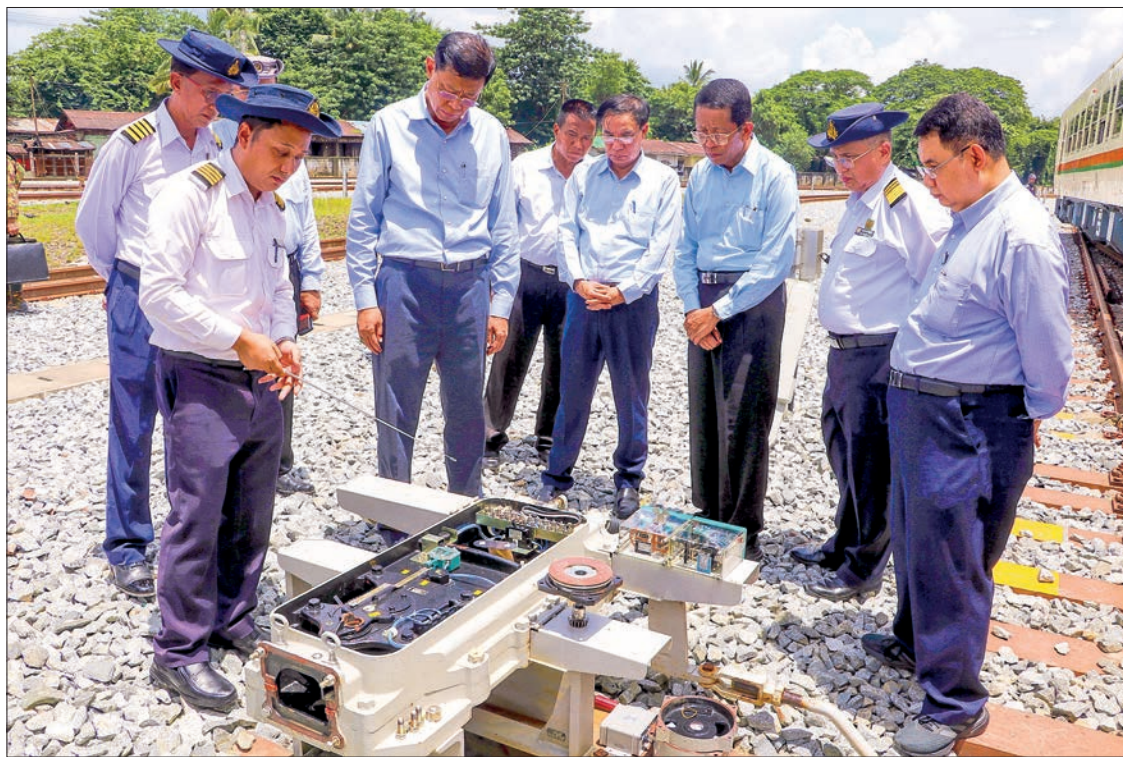
State Administration Council Member Deputy Prime Minister and Union Minister for Transport and Communications General Mya Tun Oo hears the report by an official on Electronic Interlocking System yesterday during his inspection tours in Yangon and Bago.
