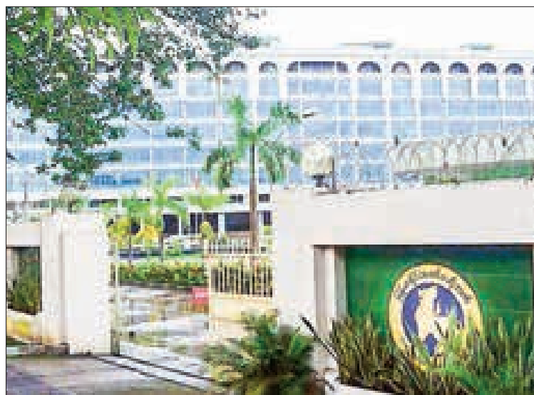
The office building of the Central Bank of Myanmar in Yangon.
