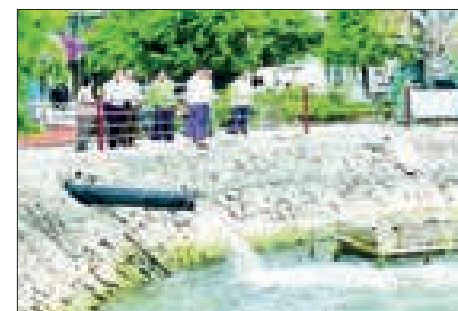
Water being pumped into Mandalay moat from a tube-well.
