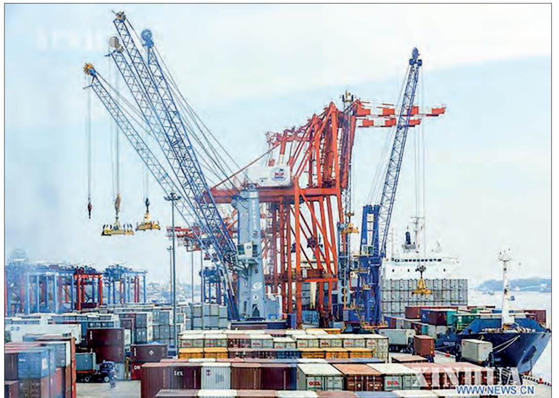
Terminal cranes are in action for loading and unloading cargo at Yangon Port.
