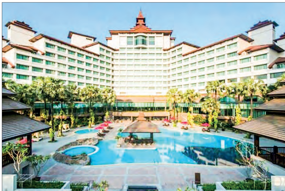
A general view of the Sedona Hotel in Yangon.
