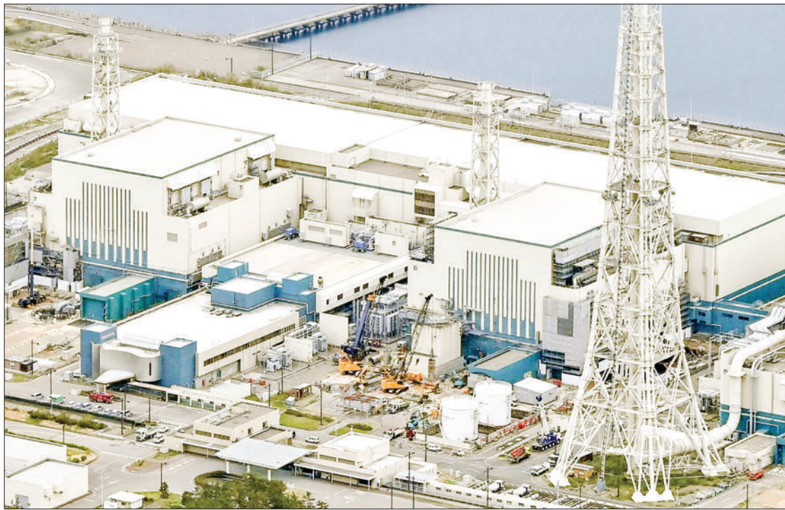
File photo taken from a Kyodo News airplane in April 2021 shows the Unit 6 (R) and 7 reactors at the Kashiwazaki-Kariwa Nuclear Power Station in Niigata Prefecture. PHOTO: KYODO
