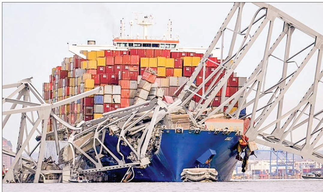
Footage of the collision showed packed container ship the Dali slamming into one of the bridge's supports, causing the 47-year-old structure to collapse. PHOTO: AFP
