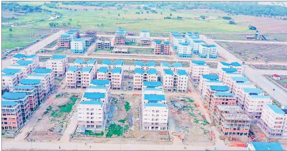
An aerial view of the new Thukha Dagon public rental housing in Dagon Myothit (South) Township, Yangon Region.
