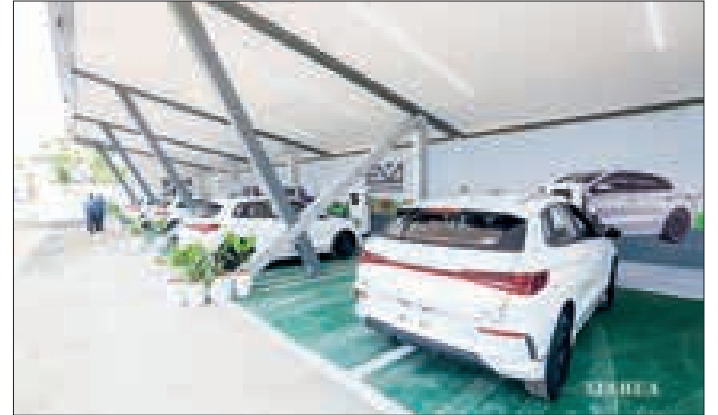
The photo depicts the first-ever EV charging station in Yangon, located in front of the Yangon Railway Station. PHOTO: XINHUA
