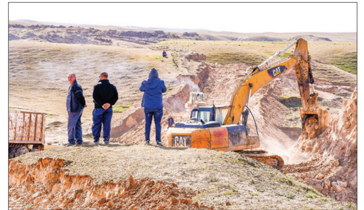
Iraqi farmers watch as excavators build up dirt barriers, a temporary measure to stem the flow of contaminated water onto farmland below, following an oil spill at agricultural land in the region of Hamrin, north of Tikrit, in the province of Salaheddin, on 19 February 2024. PHOTO: AFP
