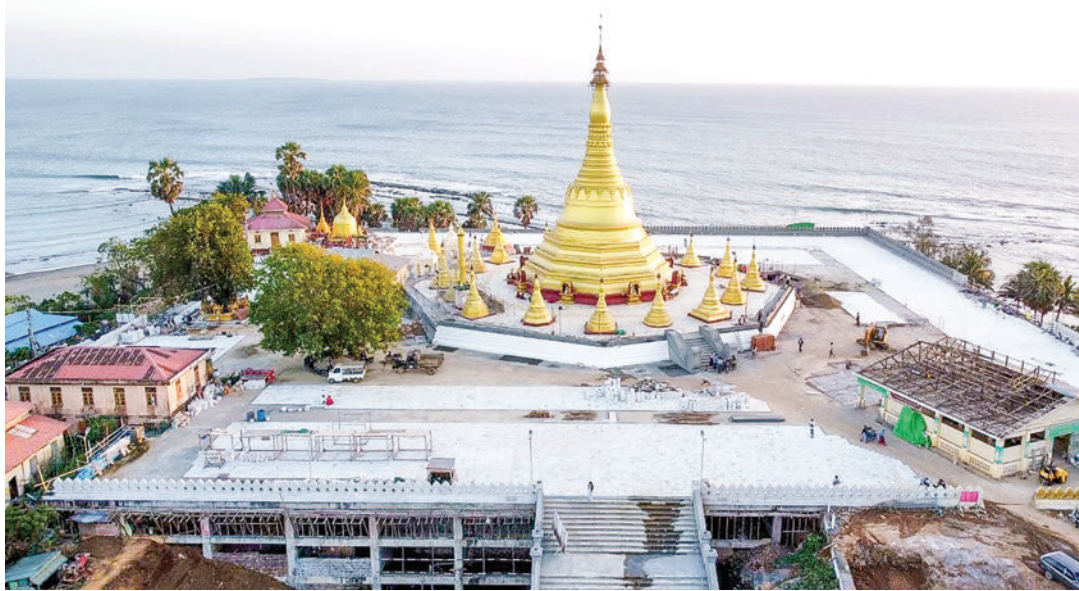
The photo shows Myat Mawtin Pagoda under renovation.
