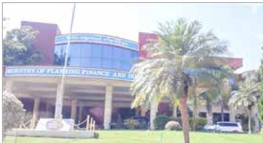
Office No 26 of the Budget Department under the Ministry of Planning and Finance in Nay Pyi Taw.
