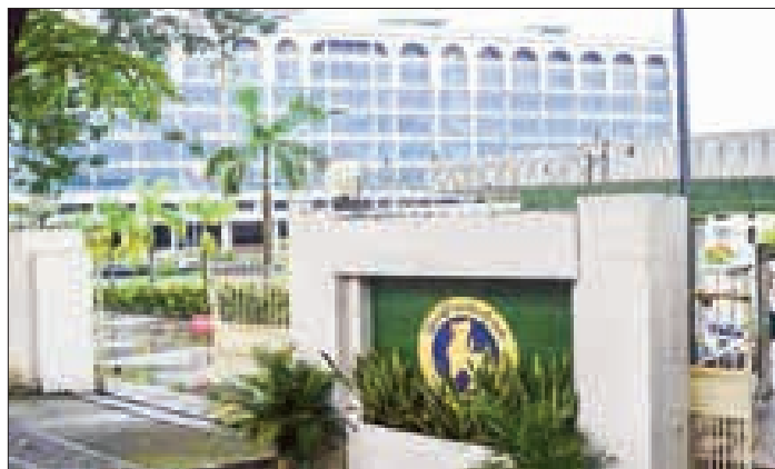
The office building of the Central Bank of Myanmar in Yangon.
