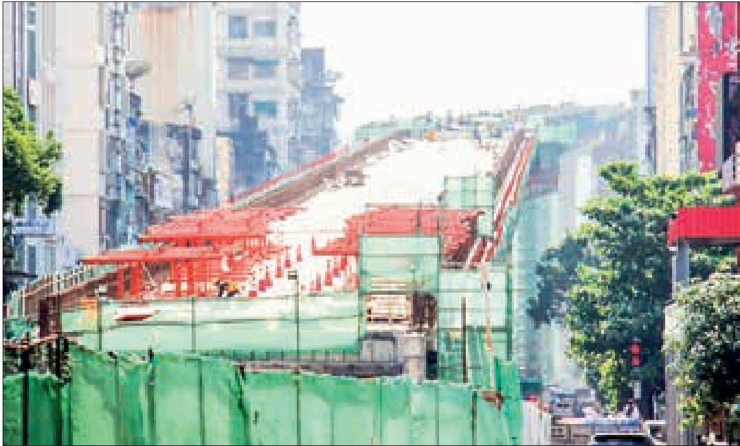
Photo shows progress of Yangon-Dala Bridge.
