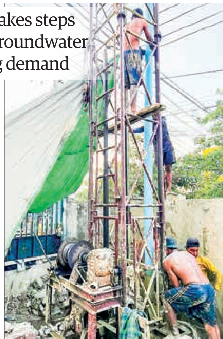
Yangon residents sinking the groundwater well.
