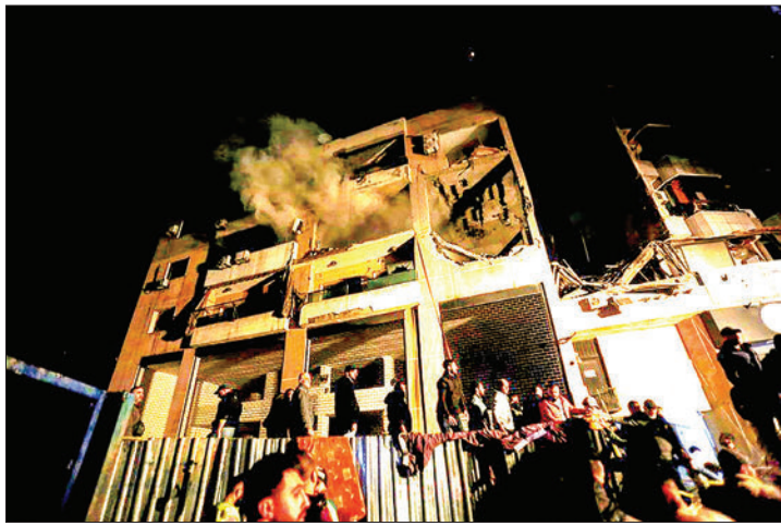
People gather outside an apartment belonging to the Hamas movement destroyed by an Israeli attack on the southern suburb of Beirut, Lebanon, on 2 January 2024. PHOTO: BILAL JAWICH/XINHUA
