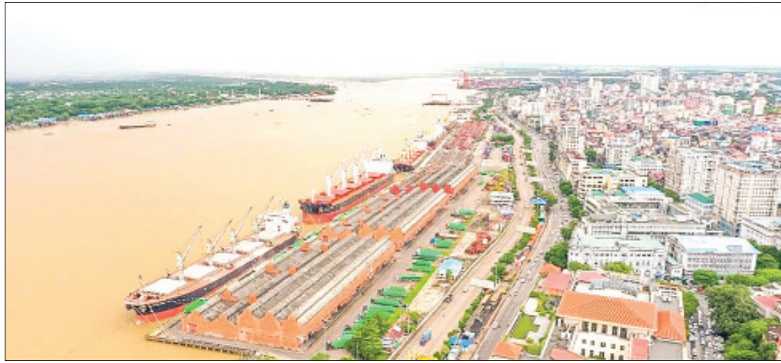
An aerial view of international port in Yangon.
