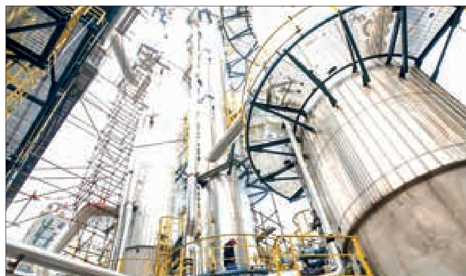
A staff member checks the ethanol production equipment with an annual output of 600,000 tonnes at Tanxin Technology Co., LTD. under the Huaibei Mining Group in Huaibei, east China's Anhui Province, 28 December 2023. PHOTO: JIN LIWANG/XINHUA
