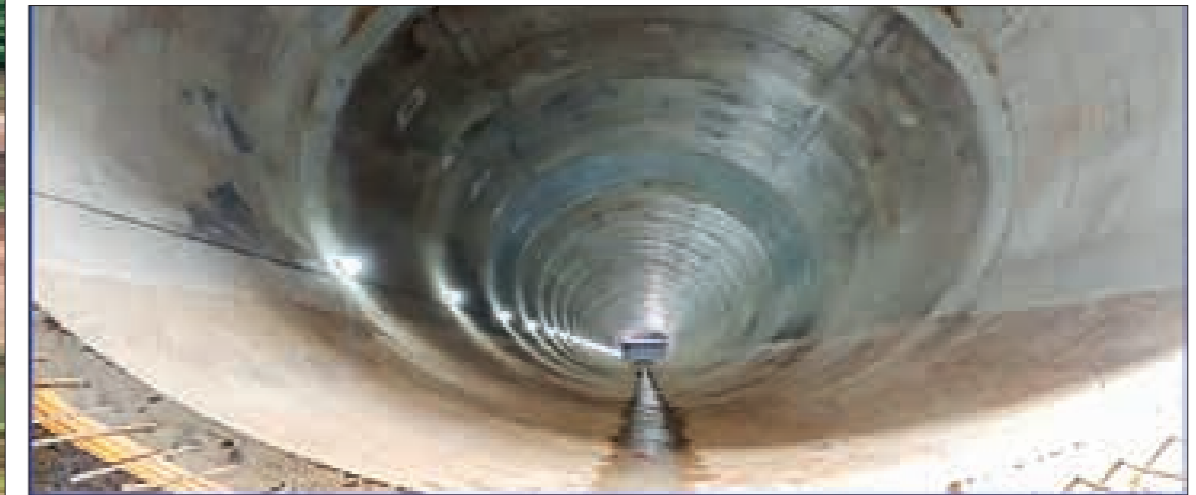
The status of underground tunnel for channeling water.
