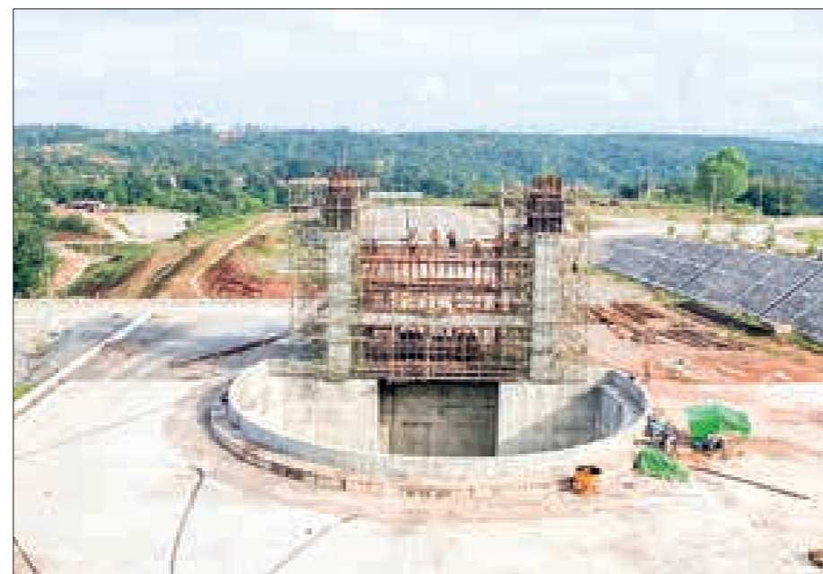
Installation of the gate to the conduit.
