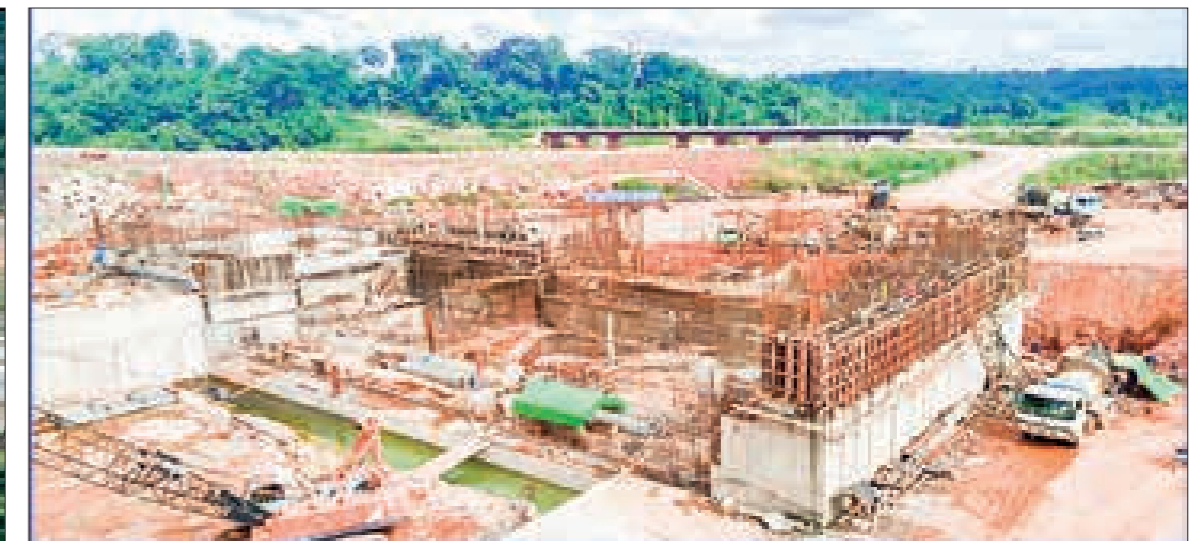
Reinforced concrete for the power station.
