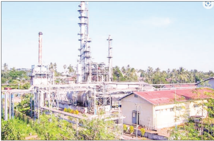
No 1 Oil Refinery (Thanlyin).
