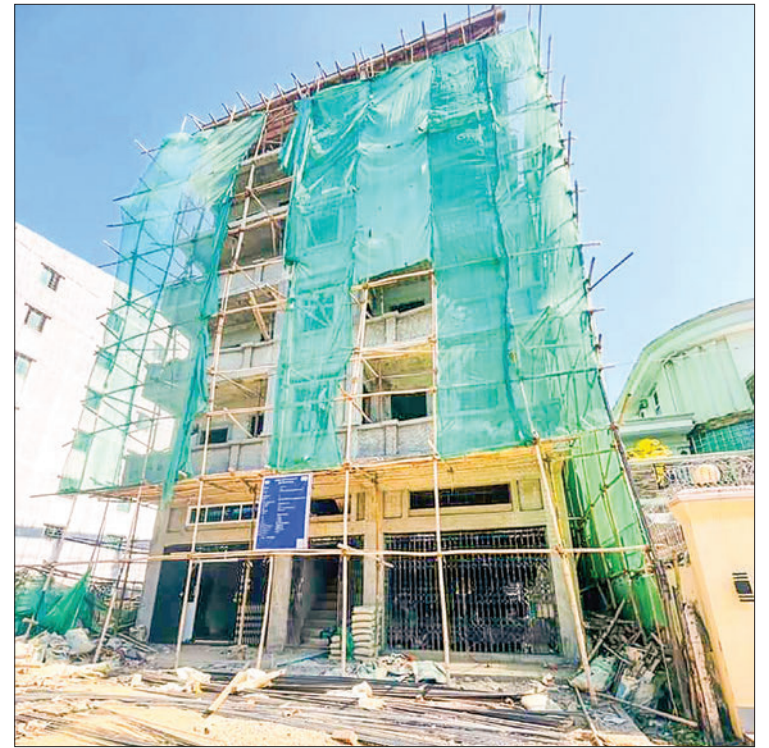
The photo shows the construction site of a building.
