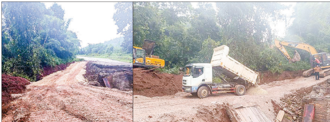
Removing measures in the Naungpit junction (L & R photos).
