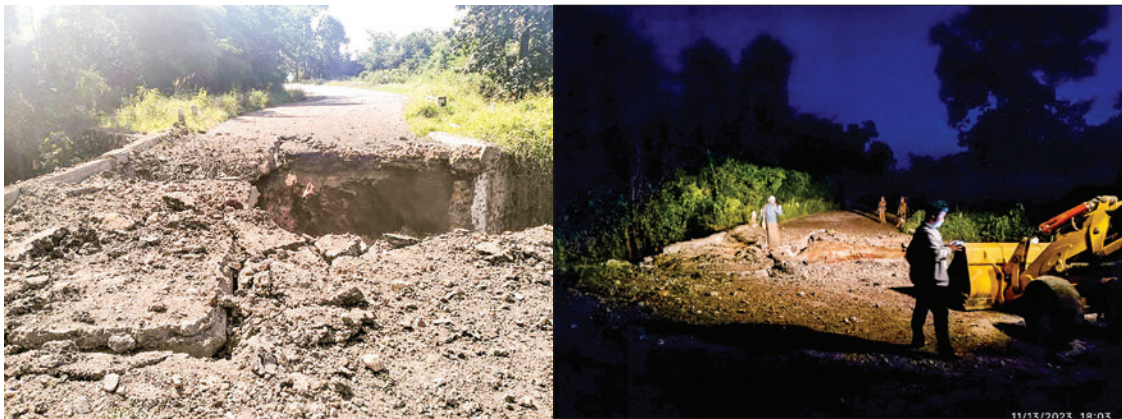
Clear-up operations in progress in Goktwin Viewpoint (L & R photos).
