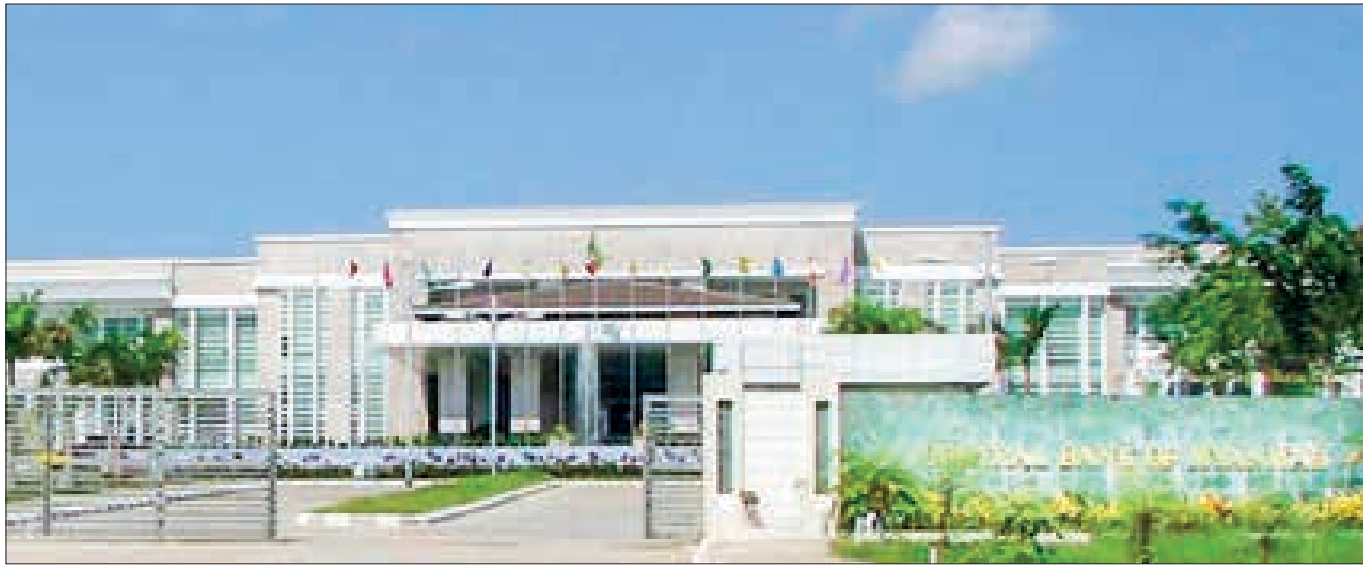
The general view of the office building of the Central Bank of Myanmar (CBM) in Nay Pyi Taw.
