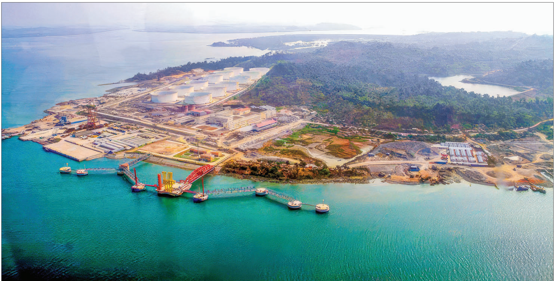
An aerial view of the Ma-de Crude Oil Discharging Terminal in Kyaukphyu Township of Rakhine State—major part of the Kyaukphyu Special Economic Zone.
