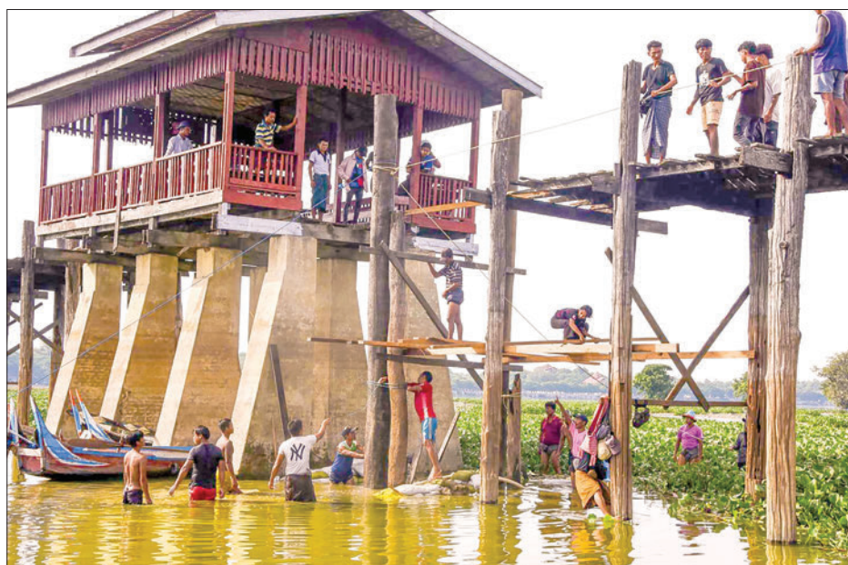
The damaged section seen under restoration.
