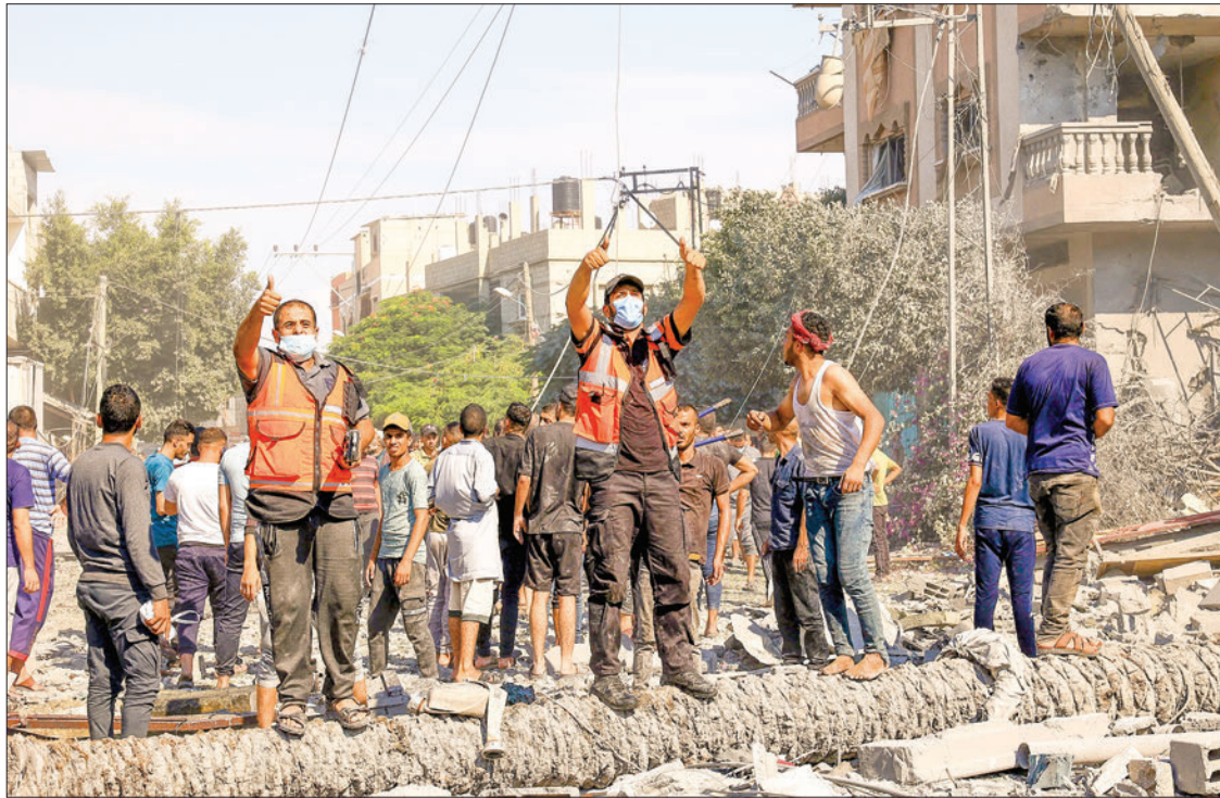
Palestinian rescuers gesture at the site of a collapsed and damaged buildings following an Israeli airstrike in Rafah in the southern of Gaza Strip on 16 October 2023. PHOTO: AFP
