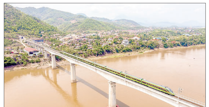
A train drives on the China-Laos Railway's Luang Prabang cross-Mekong River super major bridge in Laos 28 May 2023. PHOTO: XINHUA
