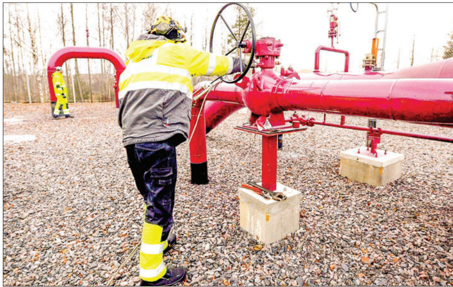
An employee operates a valve at a compression station of the Balticconnector gas pipeline between Finland and Estonia in Inkoo in 2019. PHOTO: MIKKO STIG/AFP/FILE
