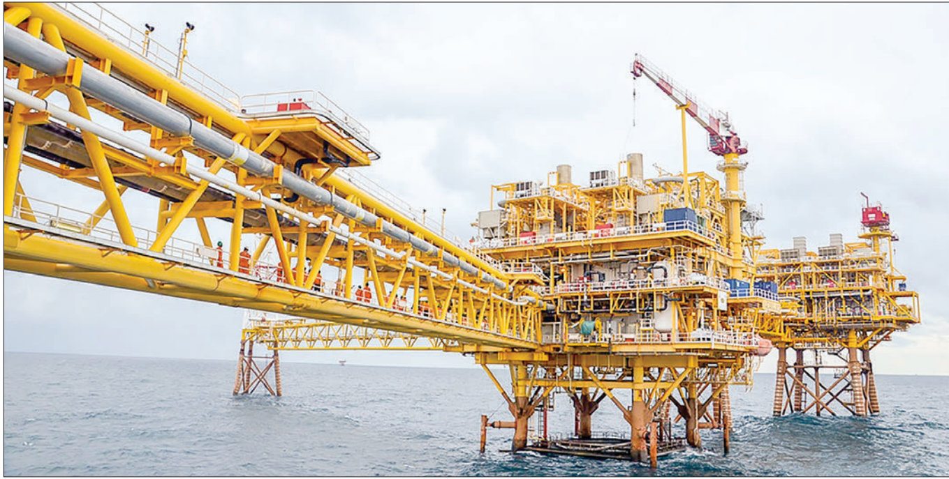
The picture depicts the Yadana Offshore Gas Platform.
