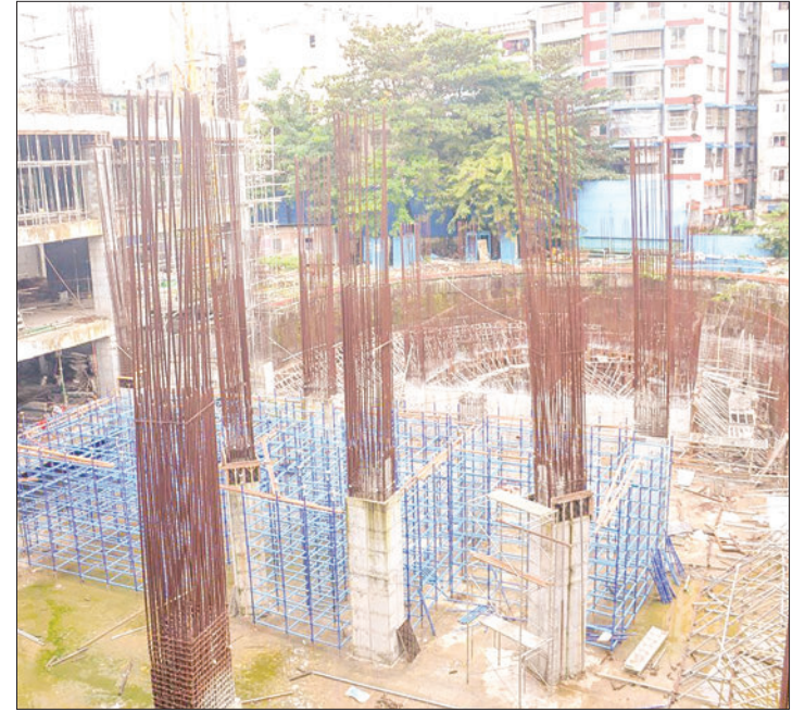
The construction site of the newly rebuilt Mingala Market.
