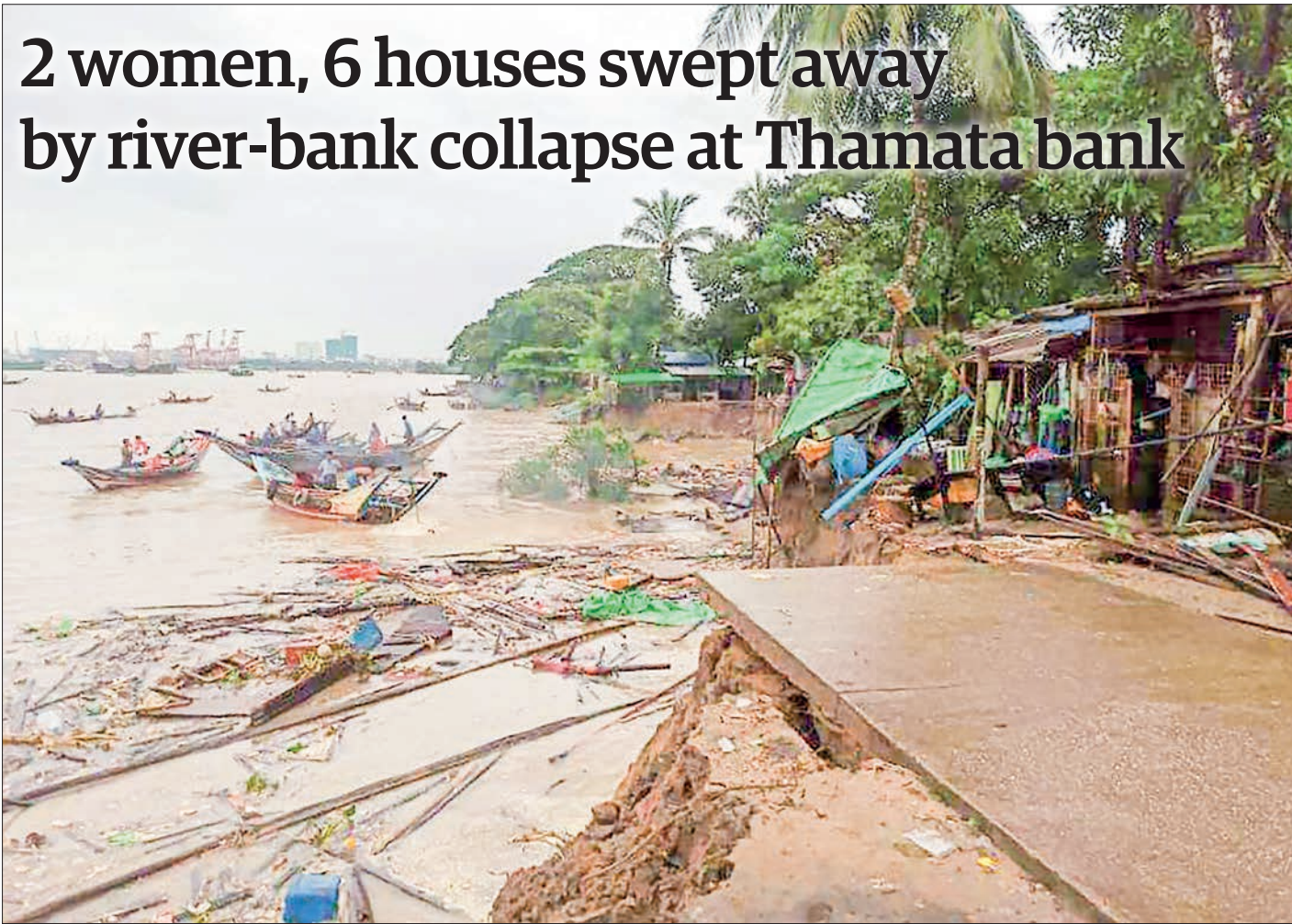
The aftermath view of a landslide incident along the Thamata bank in Dala Township.
