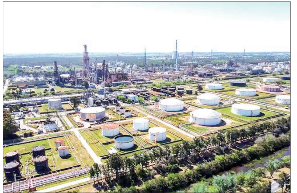
Aerial view of the Argentine state-owned oil and gas company YPF refinery in Berisso, Buenos Aires, taken on 18 October 2022. PHOTO: JUAN MABROMATA / AFP
