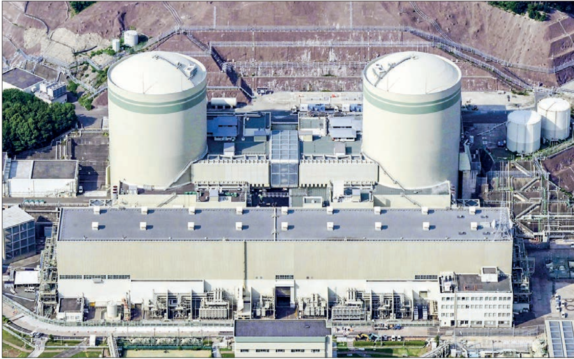
File photo taken on 28 July 2023, shows the Takahama nuclear power plant's No 2 reactor (L) and No 1 reactor in Takahama, Fukui Prefecture. PHOTO: KYODO
