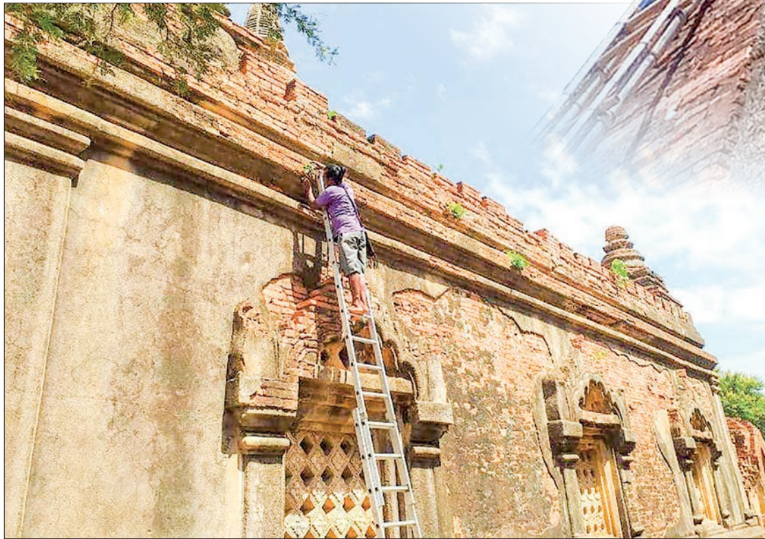
A staff from the Department of Archaeology and National Museum (Bagan Branch) removes plants on a temple of Bagan. The department cooperates with the Bagan Heritage Trust (BHT) to remove vegetation on the ancient buildings using herbicides. (above and top photos)
