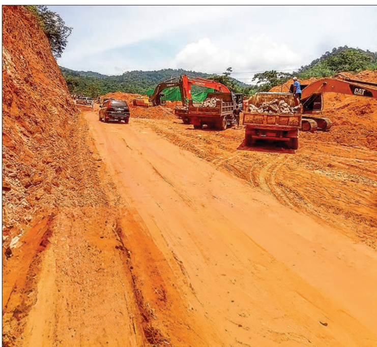
Road section undergoing repairs: Transformation in progress.
