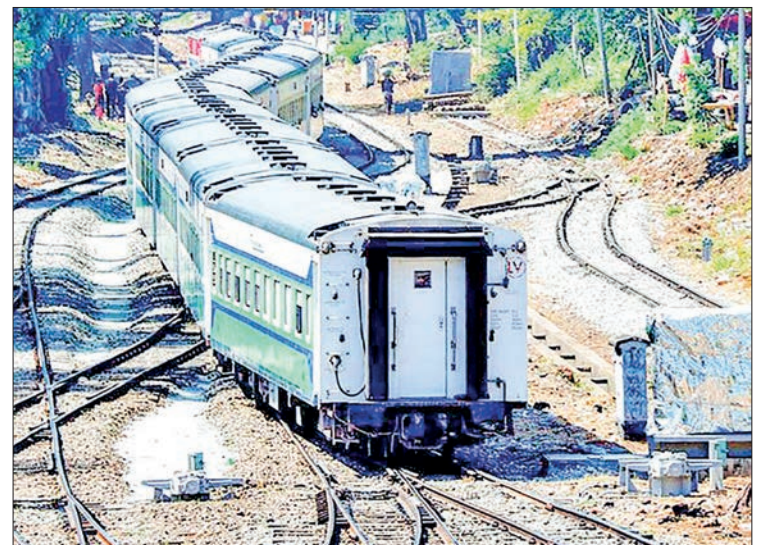
Upgrading works are seen at the Yangon Circular Rail Section.
