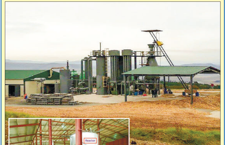
Homemade gasifier and its use for electricity generation (above and left photos.)
