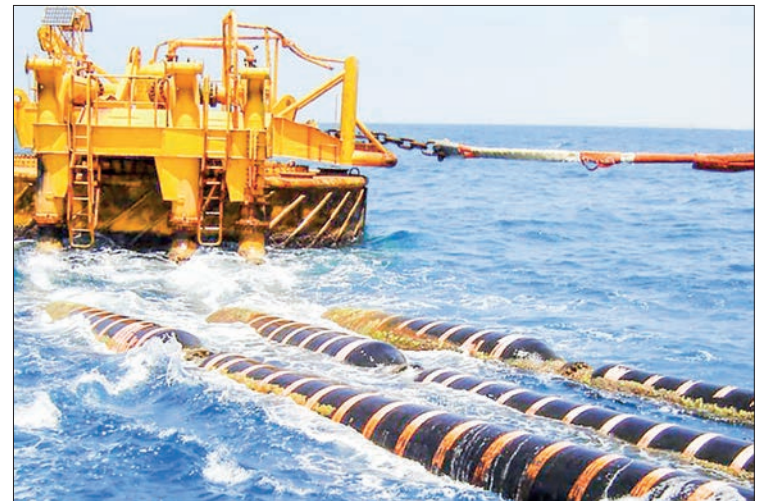
The Myanmar-Singapore international undersea cable connection project underway in Myanmar's EEZ.
