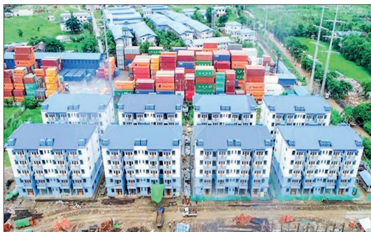
The completed apartments of Thukha Dagon Housing in Dagon Myothit (South) Township.
