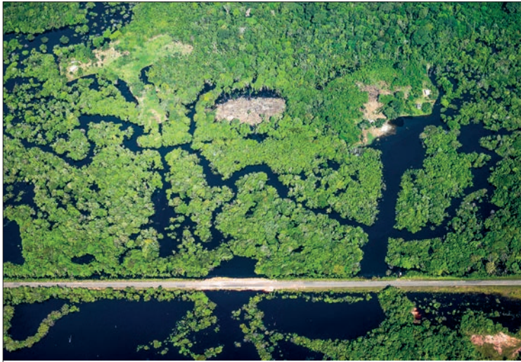
Aerial view of a road crossing the Amazon rainforest, taken from a plane flying from the city of Manicore to Manaus, Amazonas State, Brazil, on 10 June 2022. PHOTO: AFP
