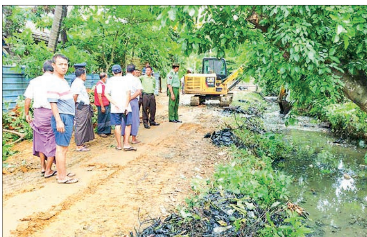
Lt-Gen Lu Aye inspects the cleaning of drainage in Kyaukpyu.
