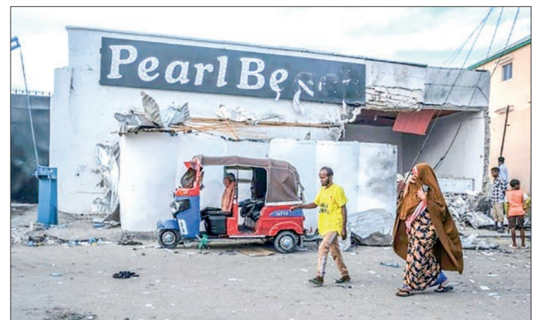
Damage after the attack at the Pearl Beach hotel and restaurant in Mogadishu PHOTO: AFP
