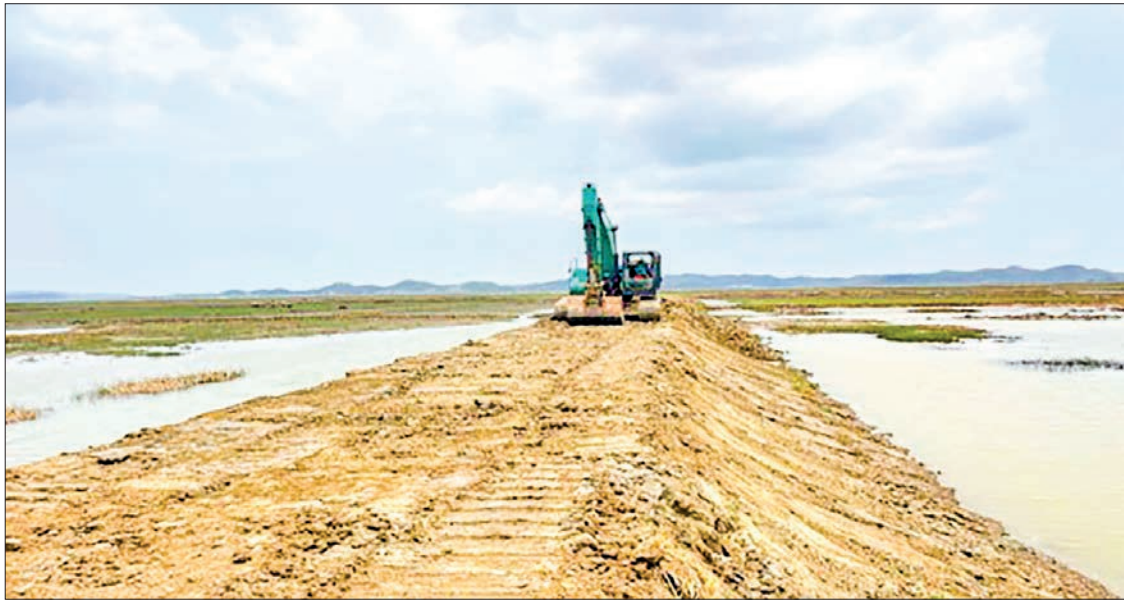
The photo shows the repair site to prevent saltwater in Sittway.
