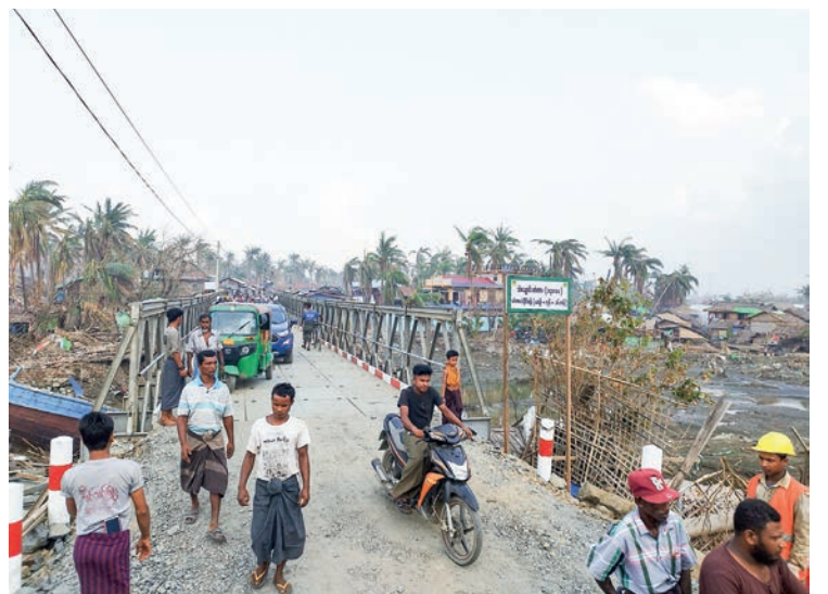
The Thechaung Bridge.
