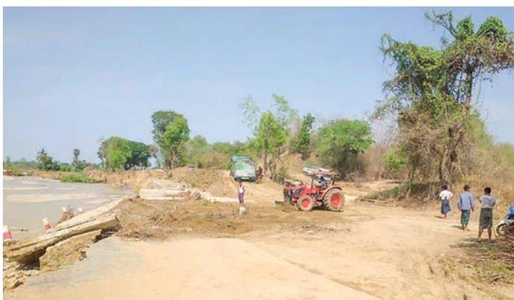
Roads eroded by Chitthaung in Seikpyu Township.
