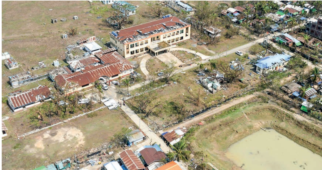
An aerial view of the damaged Township People's Hospital in Ponnagyun Township.
