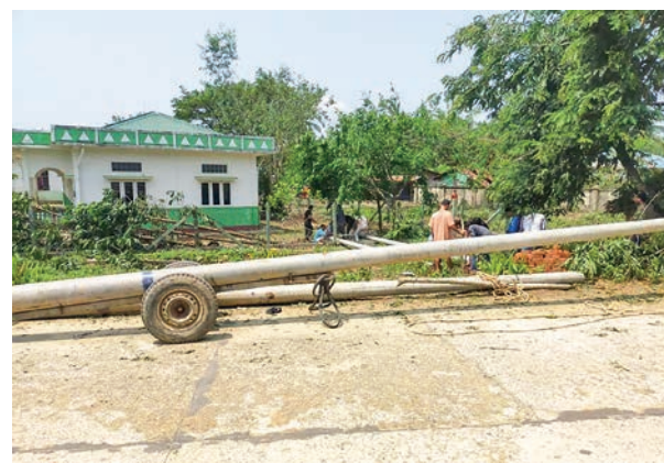
The re-erection of the fallen lamp post in Buthidaung Township.
