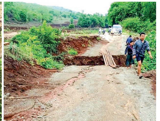
Nyaungshwe Township in Shan State.
