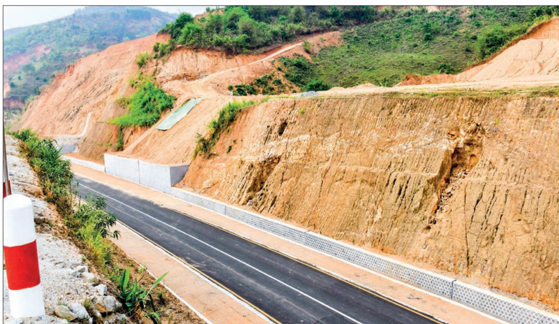
The construction site of the Kengtung detour.
