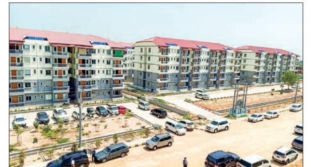
Apartments in Thukha Waddy Public Rental Housing in Dekkhinathiri Township, Nay Pyi Taw Union Territory.
